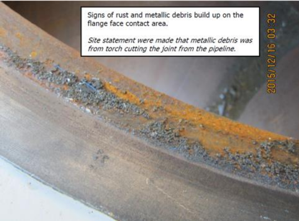
Flange with Metallic Debris
