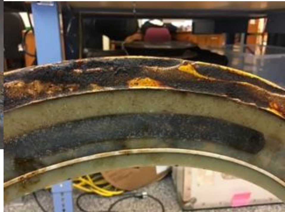
Gasket with Corrosion Residue
