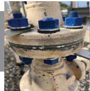
Glass Reinforced Epoxy Gasket Permeating
