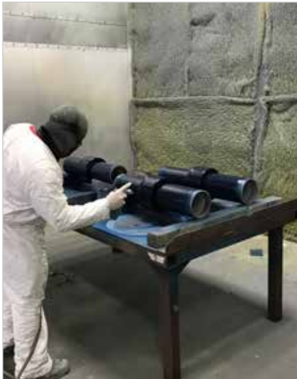
POLYURETHANE TOP COAT APPLICATION
