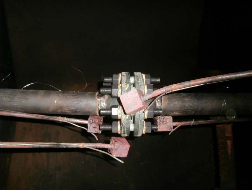
Test Setup Prior to Burn
