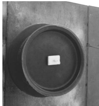
Place second cap on the sleeve and use a (block of wood*) and (wing nut*) to tighten unit in place. Make certain sleeve is plumb.
