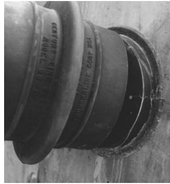
3. Place the Century-Line® Sleeve on the end cap. When field cutting non standard CS sleeve lengths, the sleeve and endcaps total length should be one-fourth (1/4") longer than the thickness of the wall.
